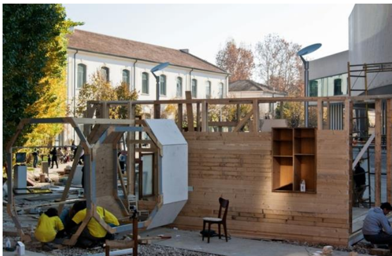
Figure 4. Day 5, The building yard
