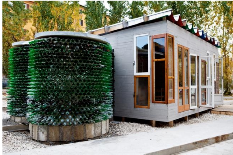
Figure 6. Day 9, Officina Roma installation is completed Note: ©Inventori di Mondì.
