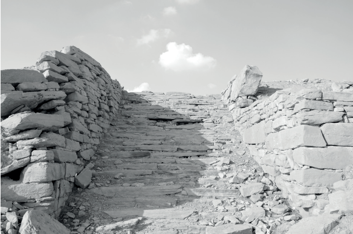
Fig. 6. The secondary stair entrance on the south side of the complex (R. Dan 2015).
