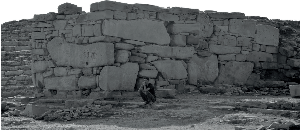
Fig. 8. The corner buttress “n”, where is well visible the different masonries used (R. Dan 2015).
