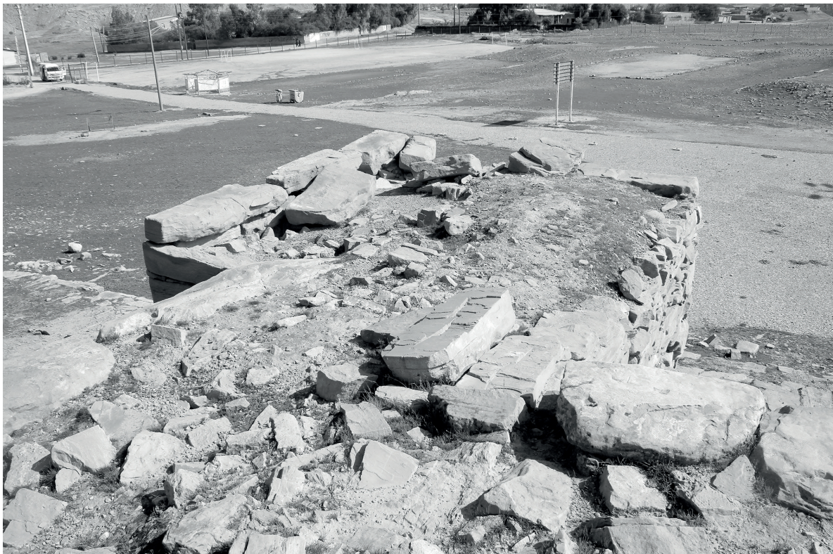
Fig. 9. The corner buttress “n” seen from the top, where is visible the filling of the terrace with loose materials (D. Salaris 2015).
