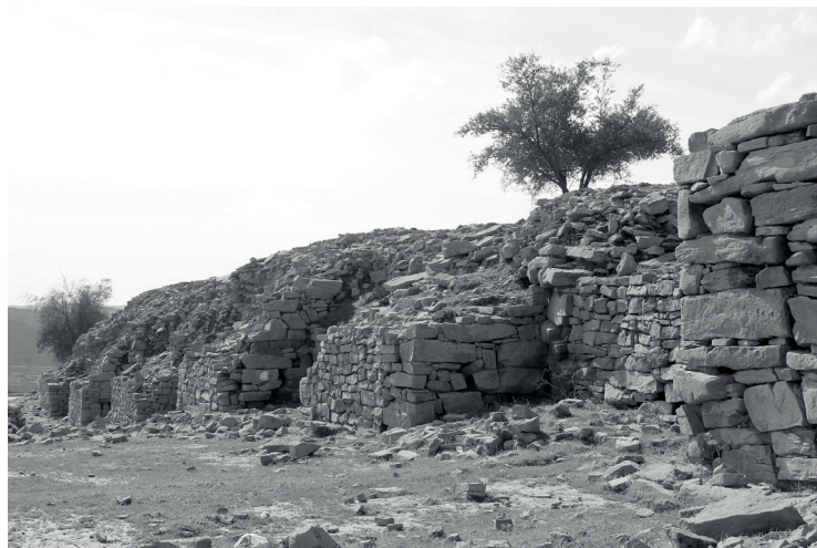
Fig. 4. The eastern retaining wall of the terrace of Masjed-e Soleyman (D. Salaris 2015).
