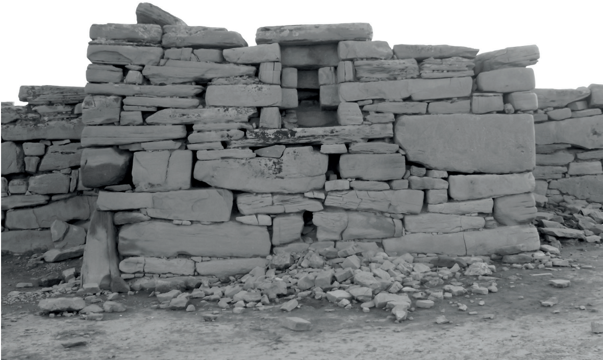
Fig. 7. The buttress “k” with one of the blind windows/niches (D. Salaris 2015).
