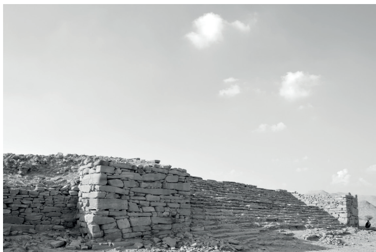
Fig. 5. The main stair entrance to the terrace (A) on the eastern side of the complex (R. Dan 2015).
