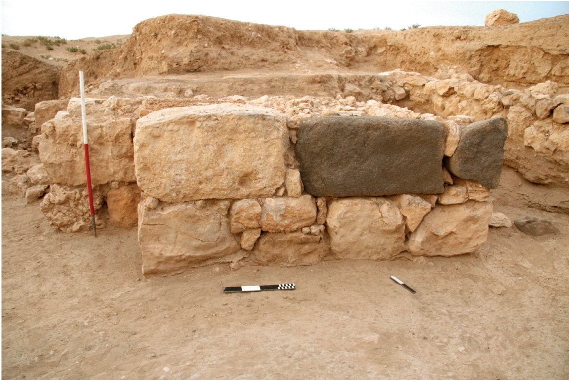
Fig. 4. Pier 500C southwest face with orthostats.
