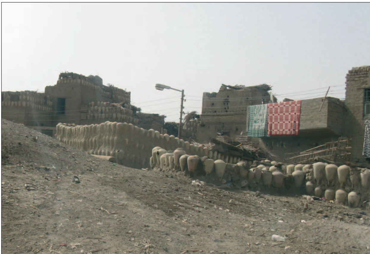
Figure 5. Walls built with pots in Naqada (Upper Egypt) (photograph by author)
