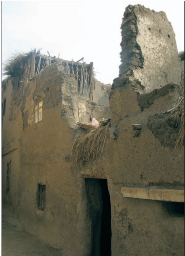
Figure 4. Collapse of upper storey structures due to lack of maintenance (Najriy, Lower Egypt) (photograph by author).
